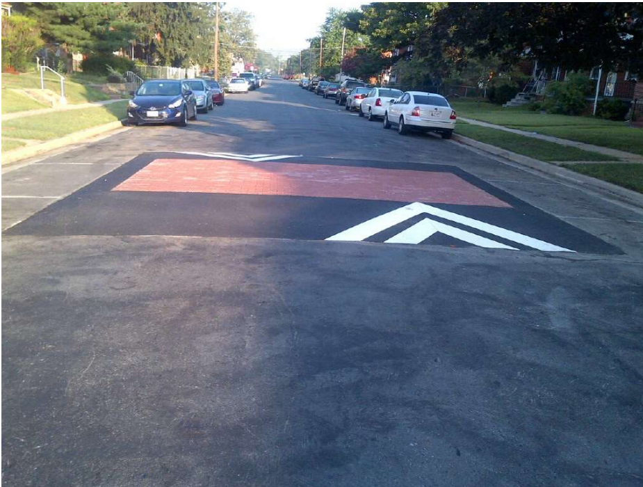
Brick top speed hump with parking on the side
