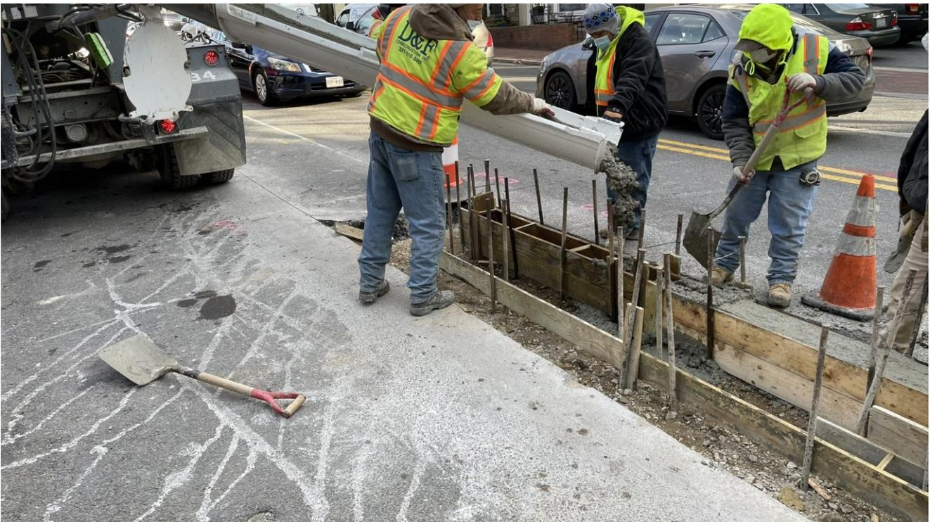
*Figure 2 - Construction of the Capital Crescent Surface Trail (CCST) in Downtown Bethesda started at the end of 2020 and will be completed in early 2021. In the photo, construction workers are building the median to separate the bike lanes from car traffic.*
